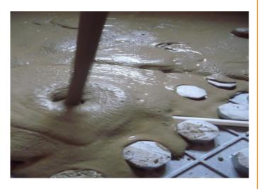
Dry and very porous substrates must be treated twice. If Casufloor C30/F6 Alpha Hemihydrate Screed is to be applied on plastic sheeting or as a floating floor, a gap of minimum 8mm should be formed around the perimeter (walls, columns, etc.)
