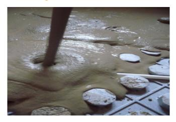
Dry and very porous substrates must be treated twice. If Casufloor C25/F5 Alpha Hemihydrate Screed is to be applied on plastic sheeting or as a floating floor, a gap of minimum 8mm should be formed around the perimeter (walls, columns, etc.)
