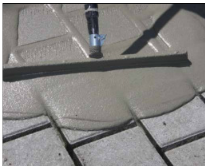
4 Filling of joints with Sopro BSF 611.
