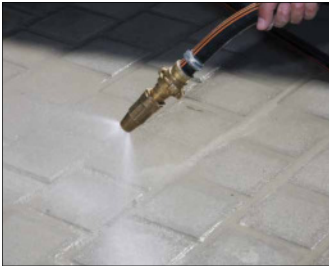
7 Spraying down with fine water spray jet after Sopro BSF 611 begins to set.
