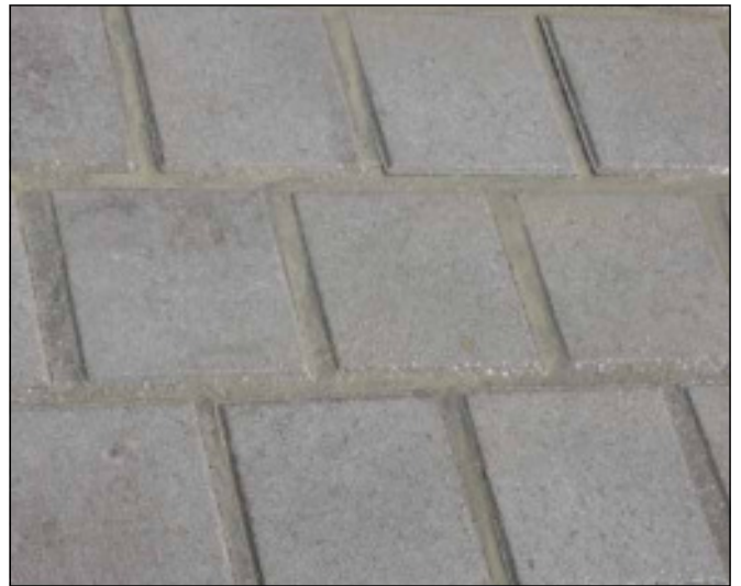
8 Grouted concrete segmental pavement.
