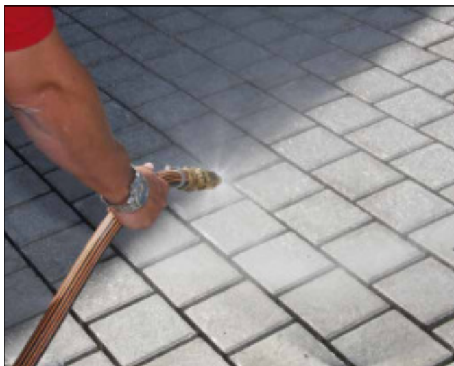
1 Pre-wetting of cleaned pavement to be grouted.
