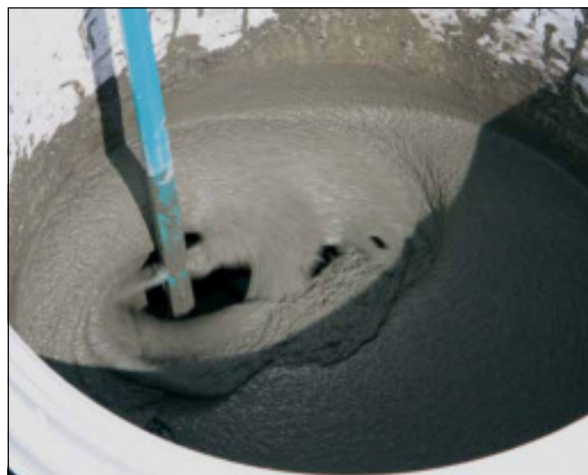
2 Preparation of Sopro BSF 611.
