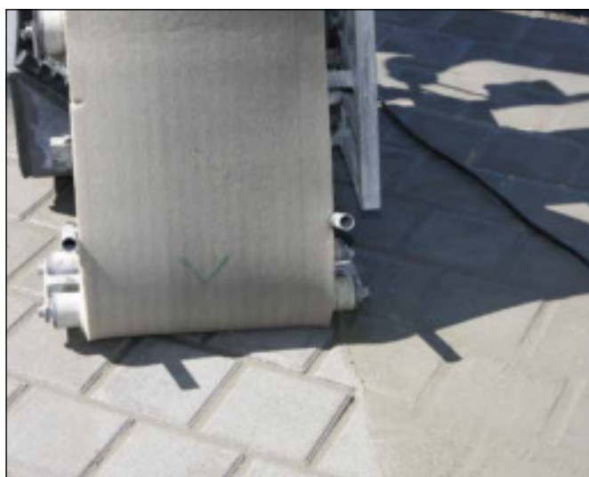
5 Washing down of pavement with cleaning machine ...
