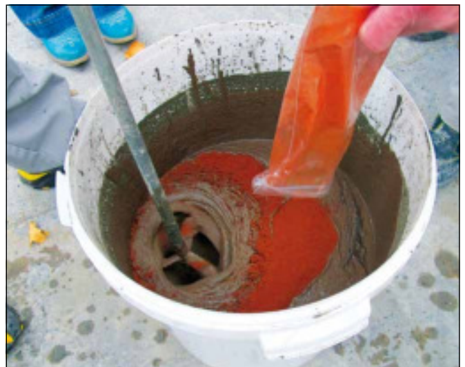
1 Addition of pigments allows preparation of grout in a variety of colours.
