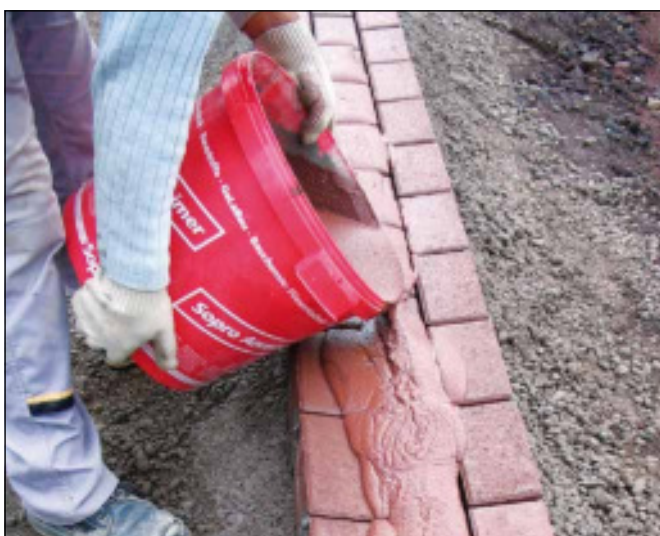
2 Application of suitably tinted Sopro BSF 611.
