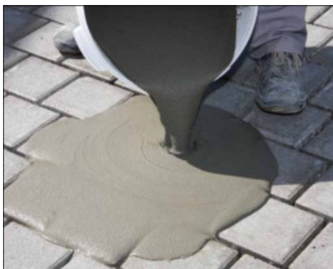
3 Pouring of Sopro BSF 611 onto pavement.
