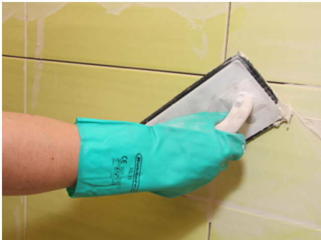
9 Grouting of earthenware tiles with Sopro DF 10 ® .
