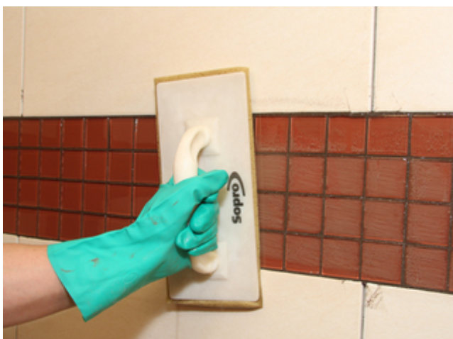
5 Allow adequate drying time for tile grout, then wash down glass mosaic.
