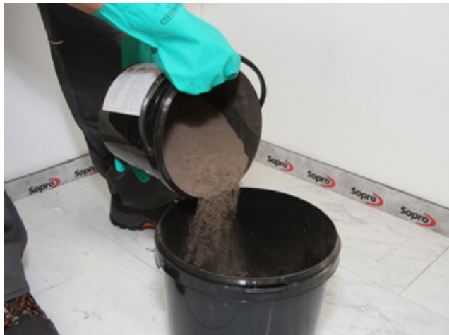
2 Add powder of Sopro DF 10 ® and mix mechanically.
